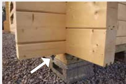
Drilled in threaded rod for wind safety
