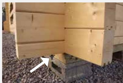
Drilled in threaded rod for wind safety
